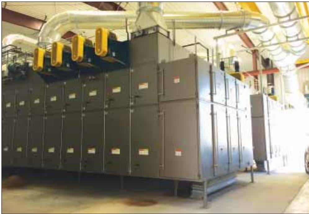
*Two Böhler Aeroglide dryers replace conventional pellet coolers at the Ainsworth mill. They are designed to increase range cube shelf life by removing all water activity. Photo courtesy of EBM Construction Inc.*
